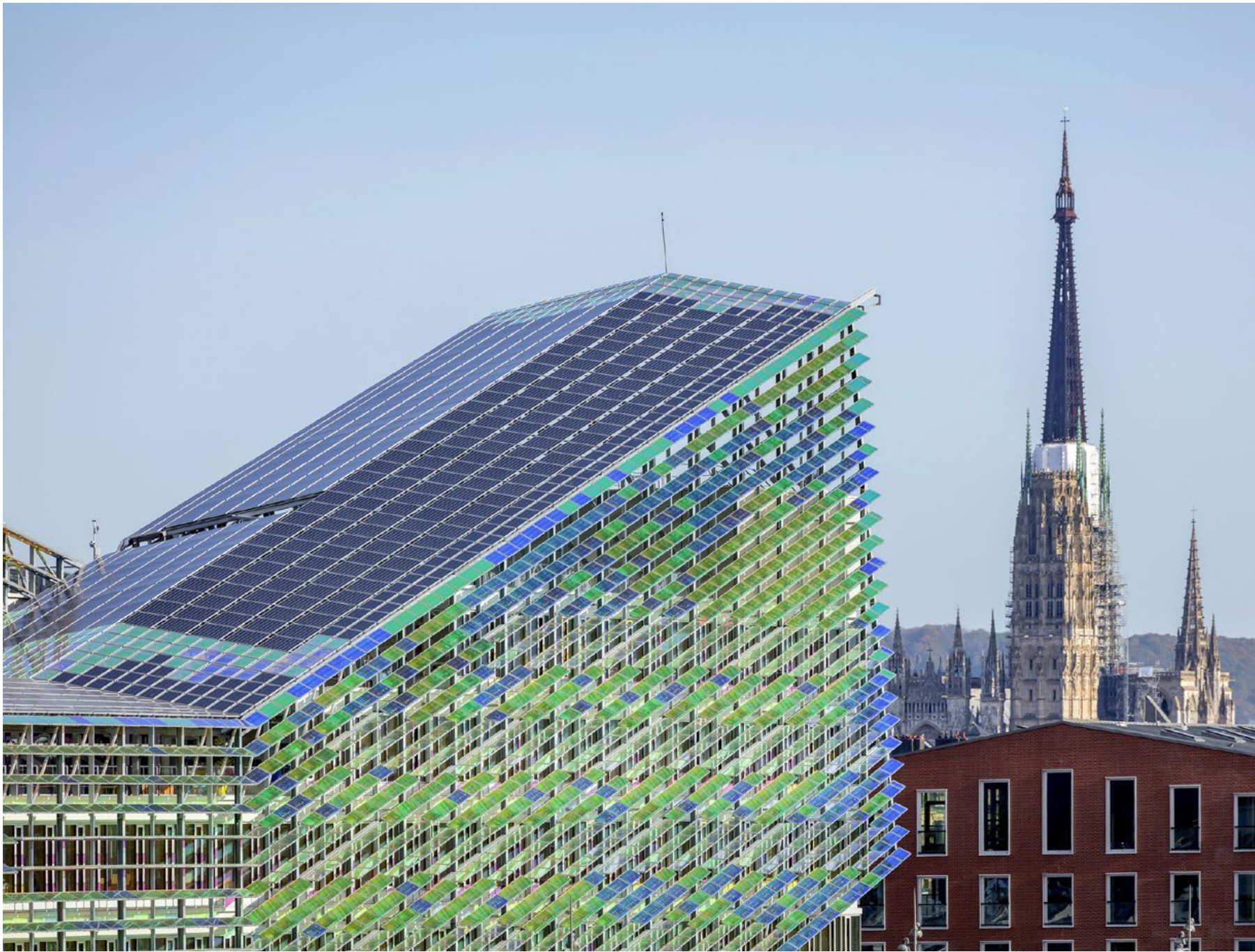
3. Métropole Rouen Normandie HQ— Integrated Photovoltaic panels on the roof and facade. Ferrier Marchetti Studio
